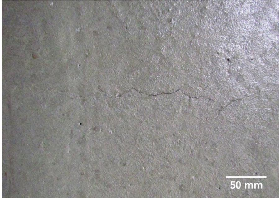
Figure 4.6: Plastic shrinkage cracking in CM
