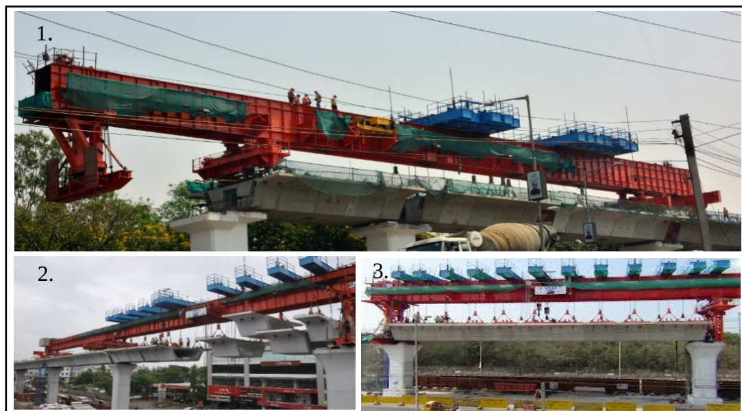
Figure 1.3: Launching girder during different operations 1. Auto Launching; 2. Segment Lifting; 3: Span Lowering
