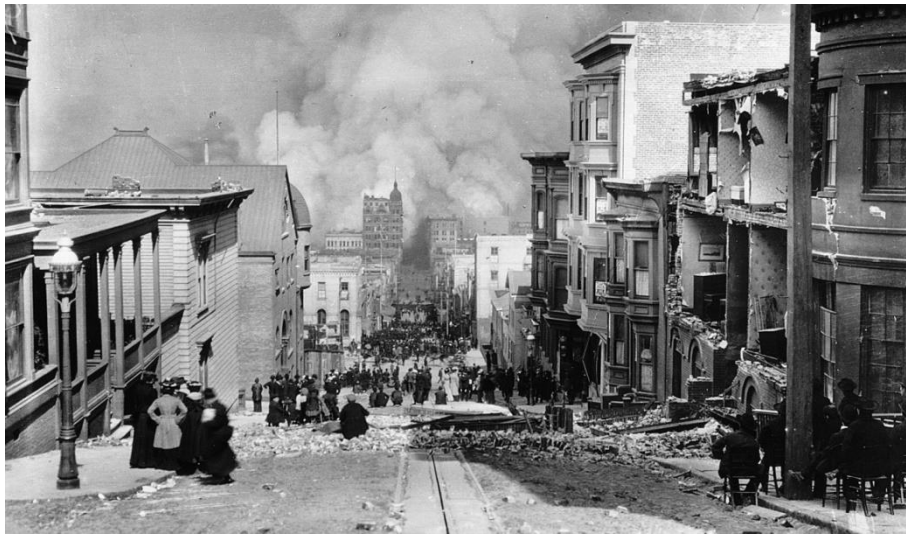
Fig. 1.2 San Francisco Earthquake damage, 1906
