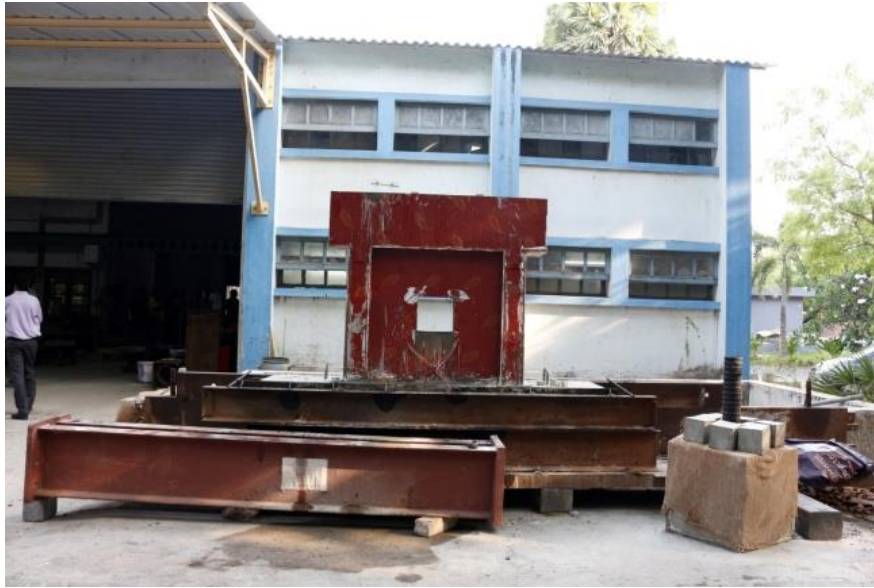
d. Preparation of wall Specimen
