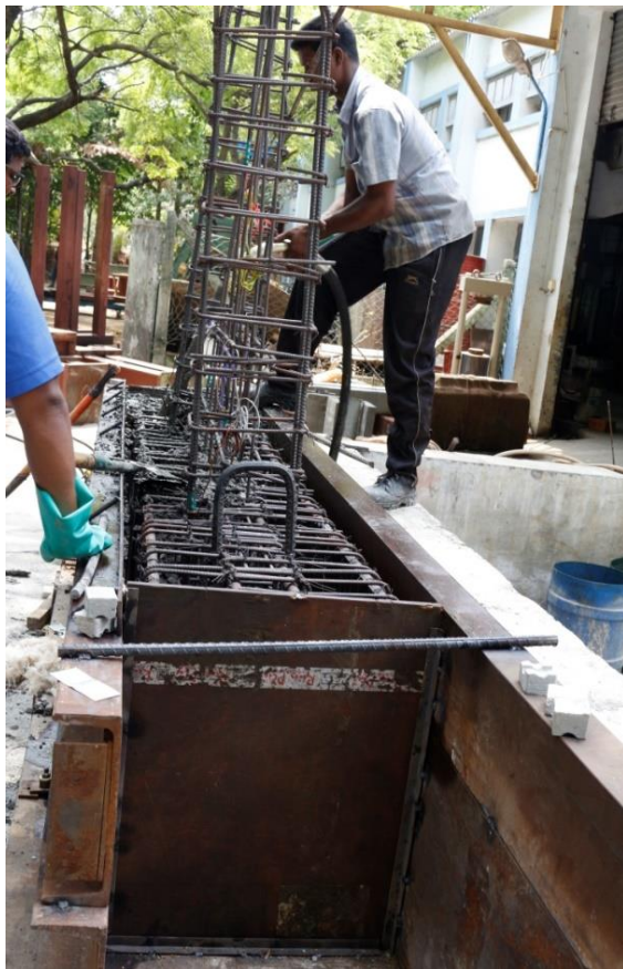
a. Concreting of Bottom Beam
