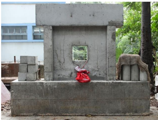
a. Wall with Window Opening
