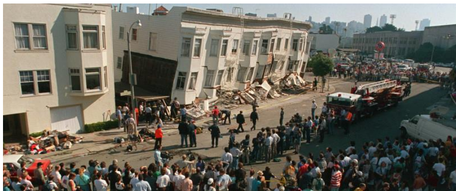
Fig. 1.3 Loma Prieta earthquake, 1989
