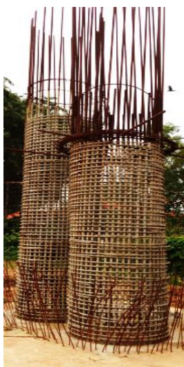
(a) Inadequate CPC coating on steel rebars used on bridge piers
