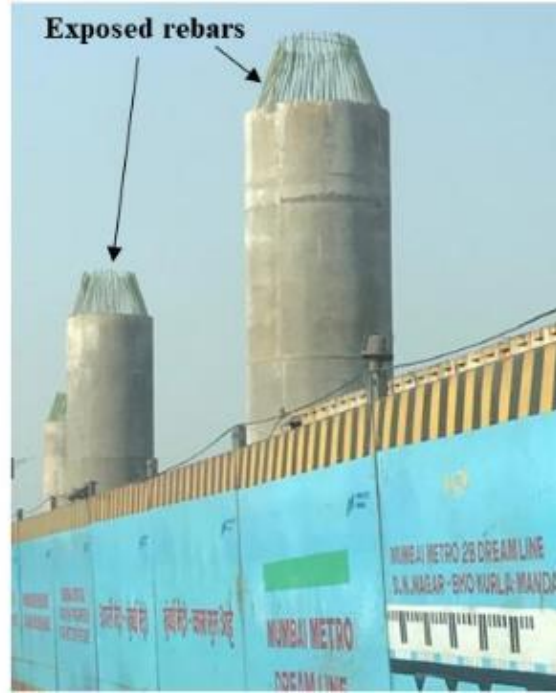
(b) Rebars exposed to sunlight at pier cap
