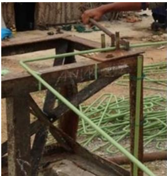
(a) FBE coated rebars are bent at a construction site using hard tools
