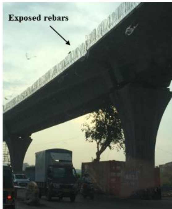
(b) Rebars exposed to sunlight at side railing
