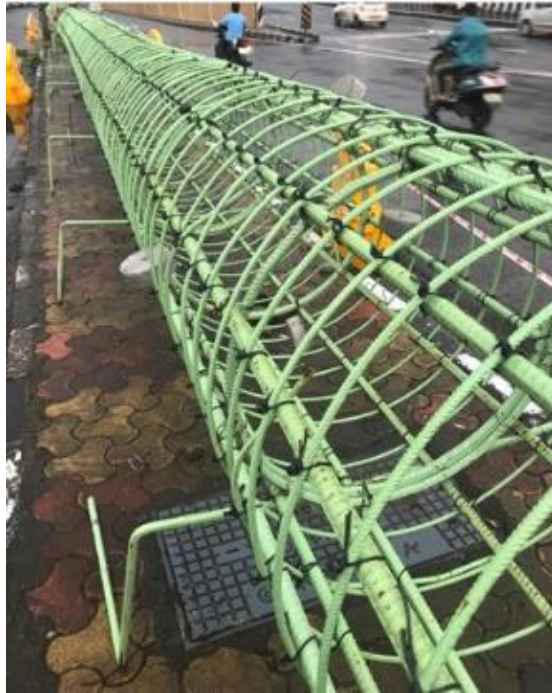
(a) Rebars exposed to sunlight during prolonged storage at construction site
