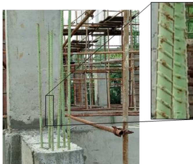
(c) Damaged coating on straight rebars during to dragging at construction sites
