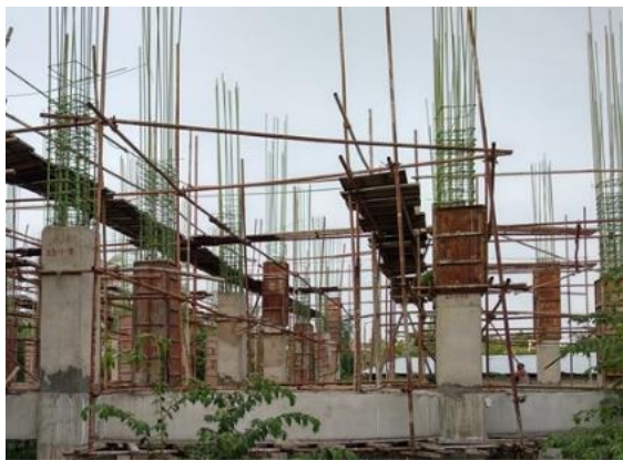
(a) Rebars used in columns
