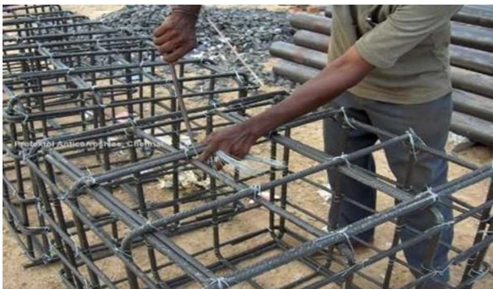
Figure 2.15 CPC Coated steel being tied by metallic uncoated tie wires (Central Electrochemical Research Institute Karaikudi 1993)
