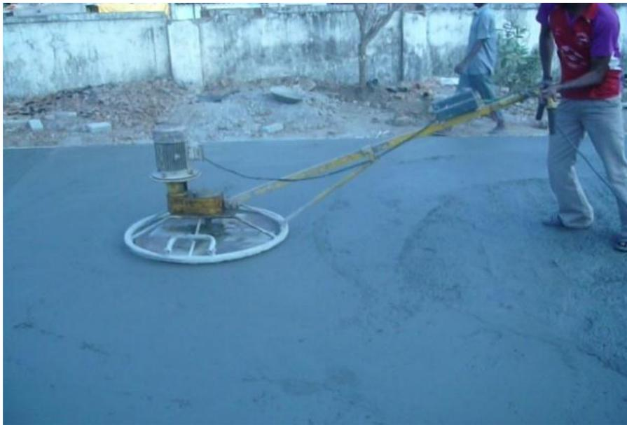
Figure 7.11 Power trowelling of freshly laid concrete surface
