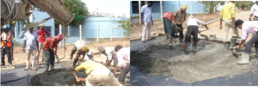
Figure 7.9 Concrete being poured and spread on the prepared surface
