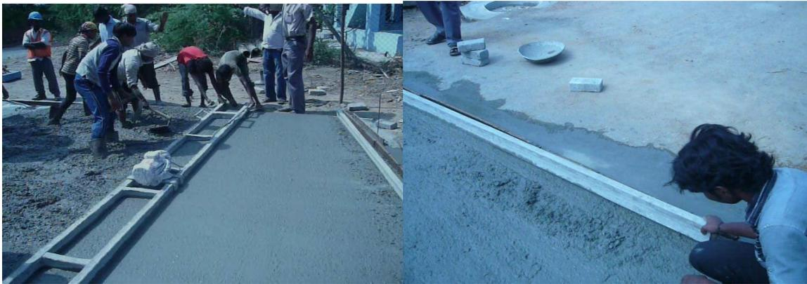
Figure 7.10 Screed vibration and manual screeding
