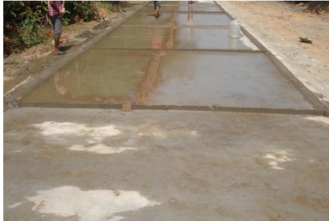
Figure 7.13 Curing of pavement surface by ponding
