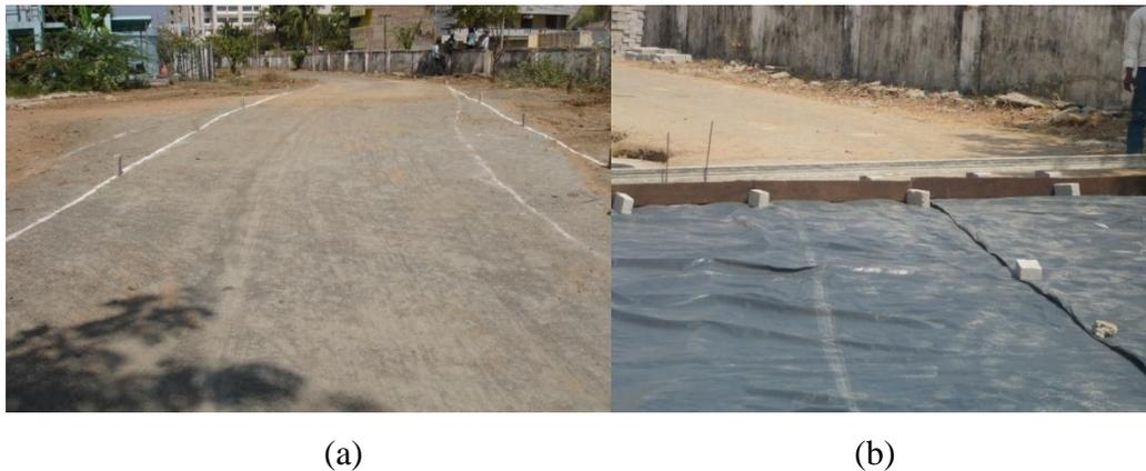
Figure 7.8 Prepared surface of the existing pavement to receive the new concrete (a) leveled surface, (b) HDPE sheet on the prepared surface
