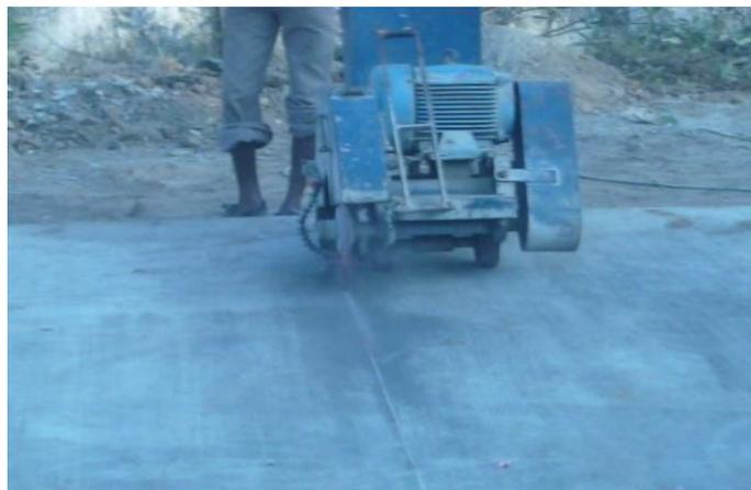
Figure 7.14 Saw cutting of grooves
