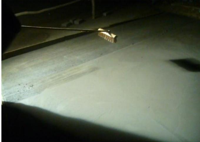
Figure 7.12 Wire brush finishing for final surface texturing
