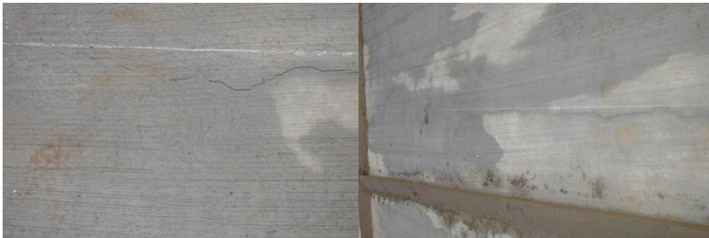
Figure 7.15 Crack occurred within 48 hours after casting during the second phase
