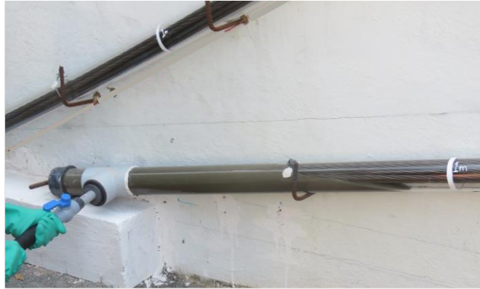
b) Injecting grout to inclined duct
