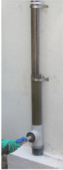
a) Pumping grout to the vertical duct
