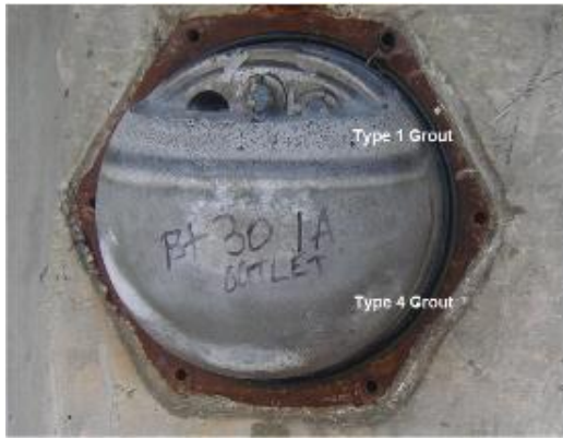
(a) A layer of softgrout on an opened anchorage zone (FHWA 2013)
