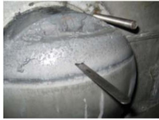
(b) A layer of highly permeable softgrout with a ruler pierced into it (FDOT 2016)
