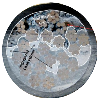
a) Cross-section of segregated grout
