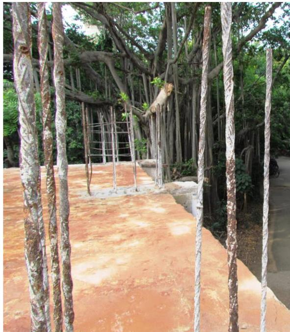
Figure 3.4 The extender rebars (corroded CTD steel rebars) used in the dummy columns on top of the roof slab of the building
