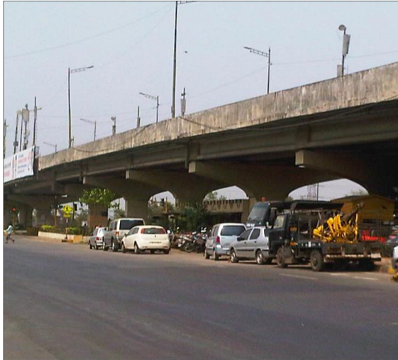
(a) A pretensioned concrete bridge on an elevated highway
