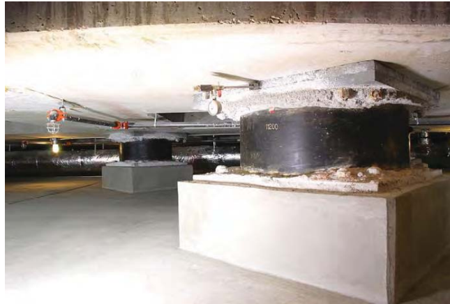
Figure 1.6 Typical base isolation below buildings(source: https://en.wikipedia.org/wiki/Base_isolation )
