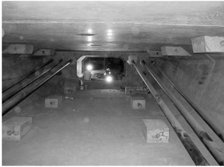
**Fig. 1.** Typical interior view of box girders in PT bridges (six external tendons are visible)
