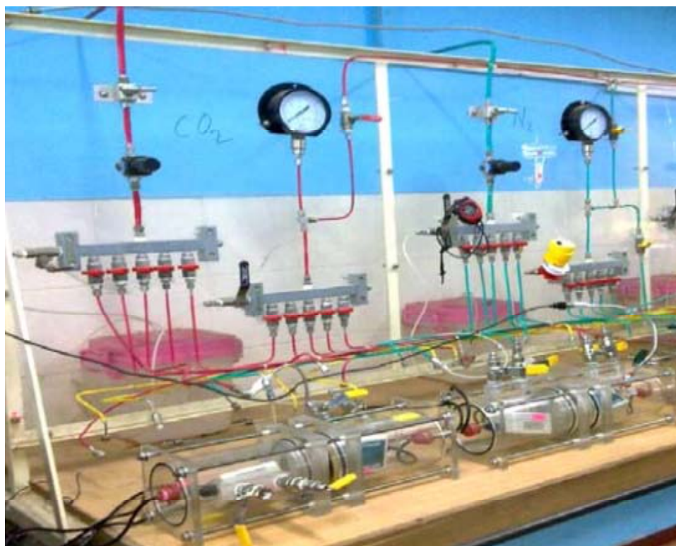
Figure 3.20 Gas distribution and pressure control panel
