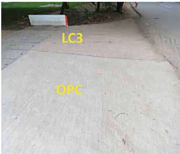
(c) Integrity of pavement segments in September 2019.
