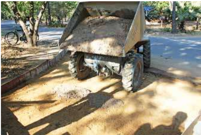
(a) Concrete pour for a pavement segment with FRC made with LC 3 .
