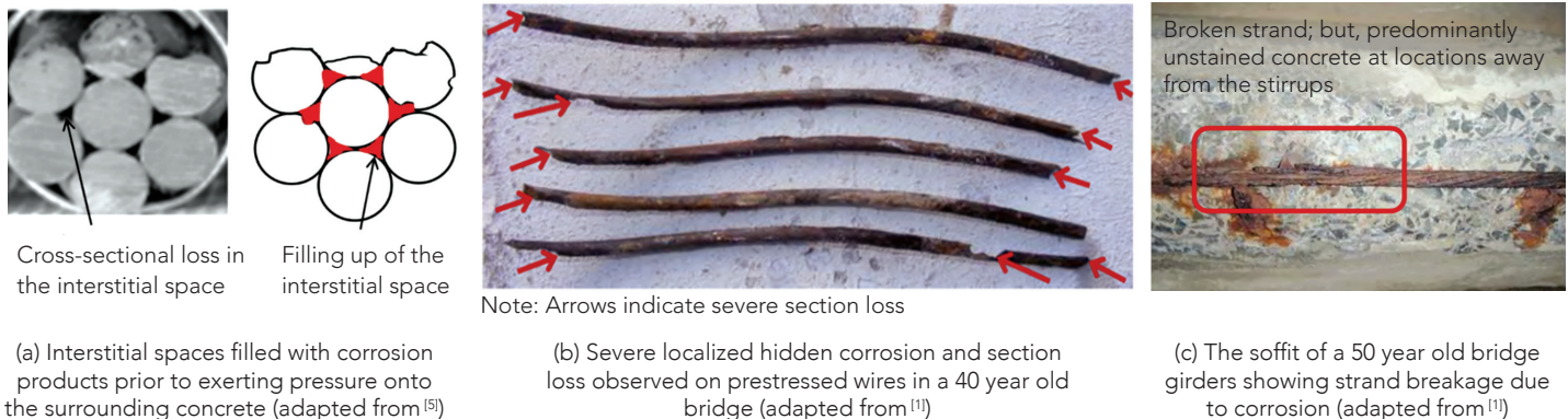
Figure 1: Insidious and hidden nature of strand corrosion in PTC systems
