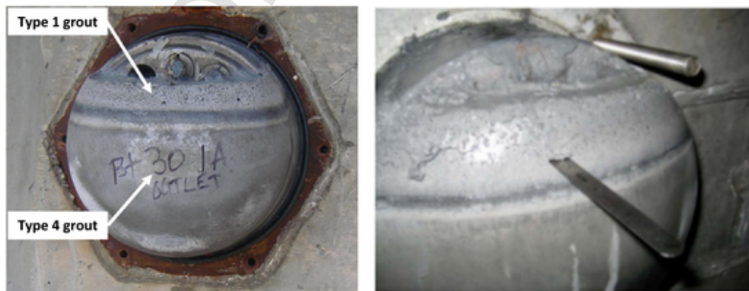
a) Opened anchorage end (adapted from [18])
